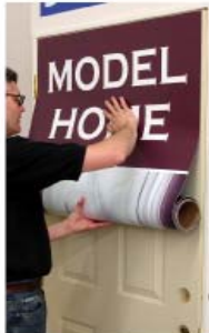
Door Protector Being Installed
